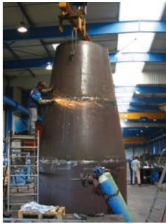
↑ Production of an aggregate storage hopper
