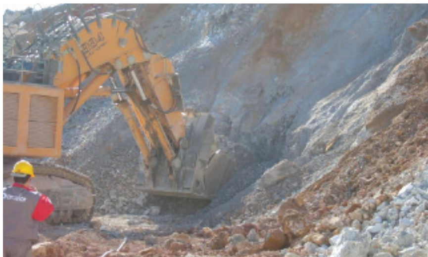
Test mining excavator bucket in use at the work face on a Liebherr ER 994B excavator
