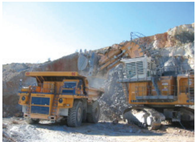
Digging with the test buckets at the work face and unloading excavated material into the dumptruck
